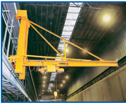
A Spanco 5-Ton Wall-Traveling Jib Crane is installed beneath an existing overhead bridge crane and covers the entire length of the facility.
